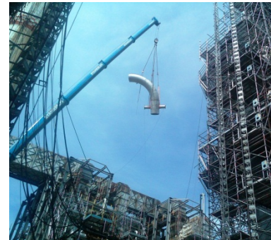
Petrobrazí shutdown impressions: 52in transfer line fit up
