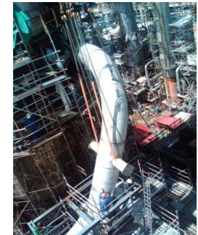
Petrobrazí shutdown impressions: 52in transfer line fit up
