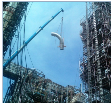
Picture: 52 inch transfer line change from 2x 24 inch; prior to CDU revamp
