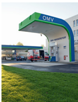
Austria's first public hydrogen filling station in Vienna.
