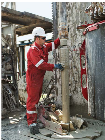
Drilling rig Erdpress, Austria
