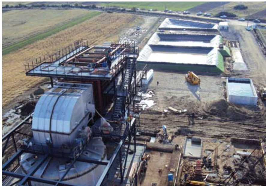
Construction of the treatment station for sludge, water, and soil
