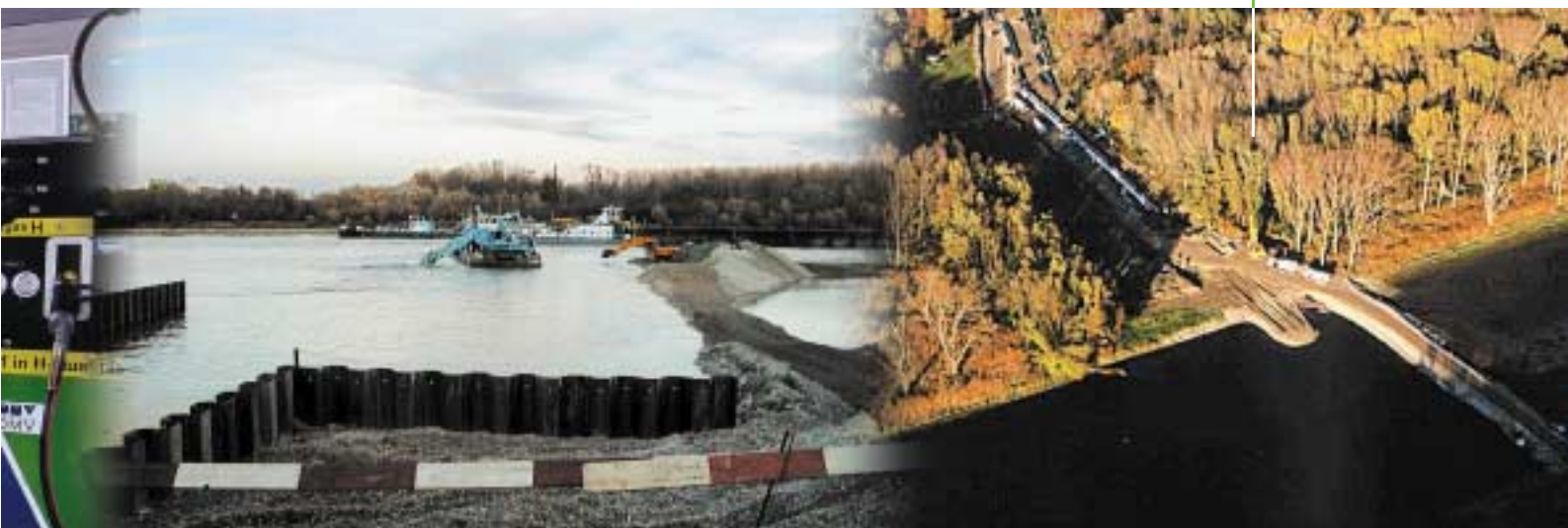
TAG Loop II, laying a gas pipeline under the Danube river
